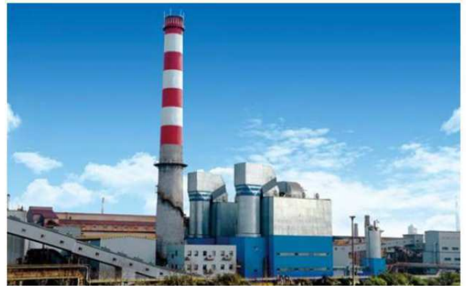
World's largest sintering machine dry FGD system for Baosteel
