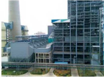
Flue Gas Denitration Device of 2×1000MW Unit in Hongshan Coal Power Plant
